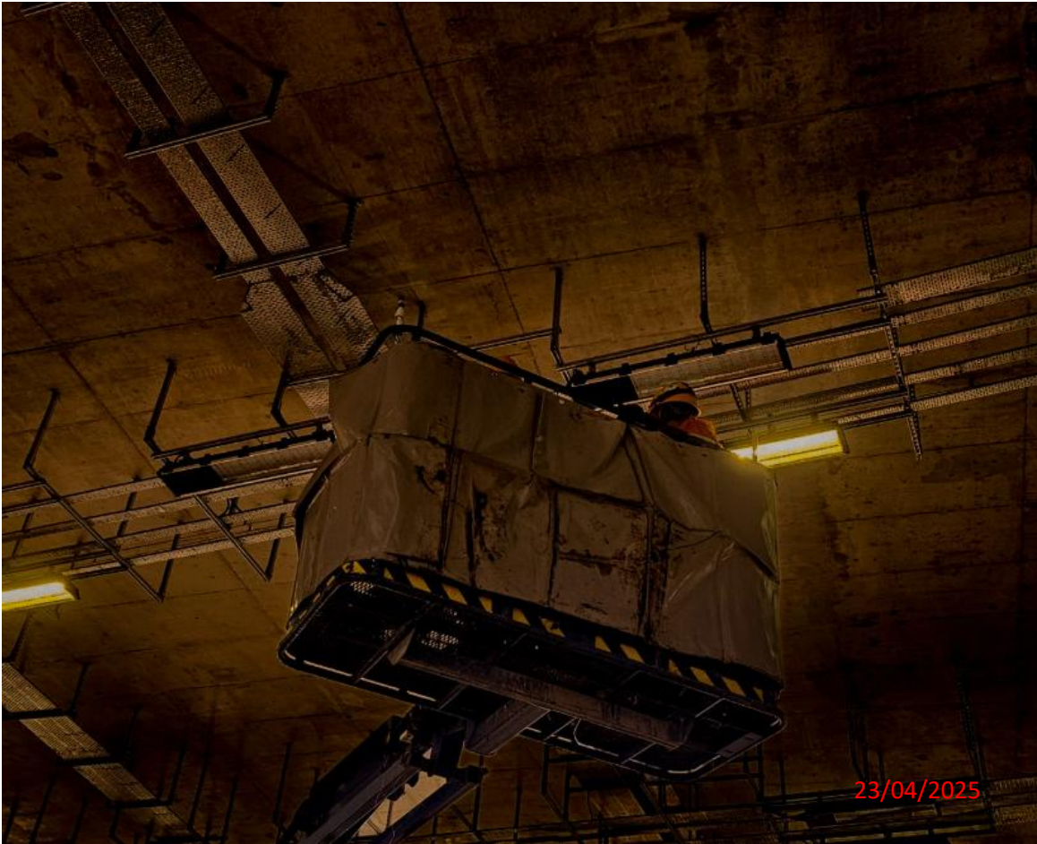
Remark 3: Site photo of noise mitigation measure
